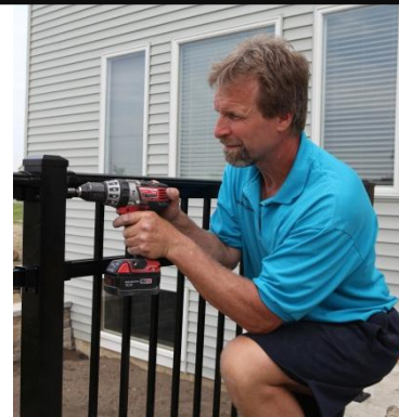
Installation Spindle – is screwed to post; best option when no angles are involved.
